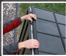
Push back roof cover to reveal tiles.
